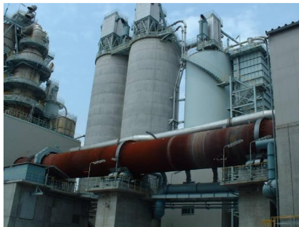
Figure 1. Ecocement plant under operation in Chiba, Japan.
