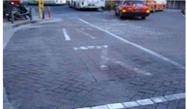
Figure 3. Sound condition at bus station.
