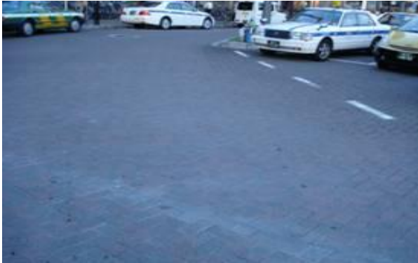
Figure 2. Sound condition at entrance and corner.
